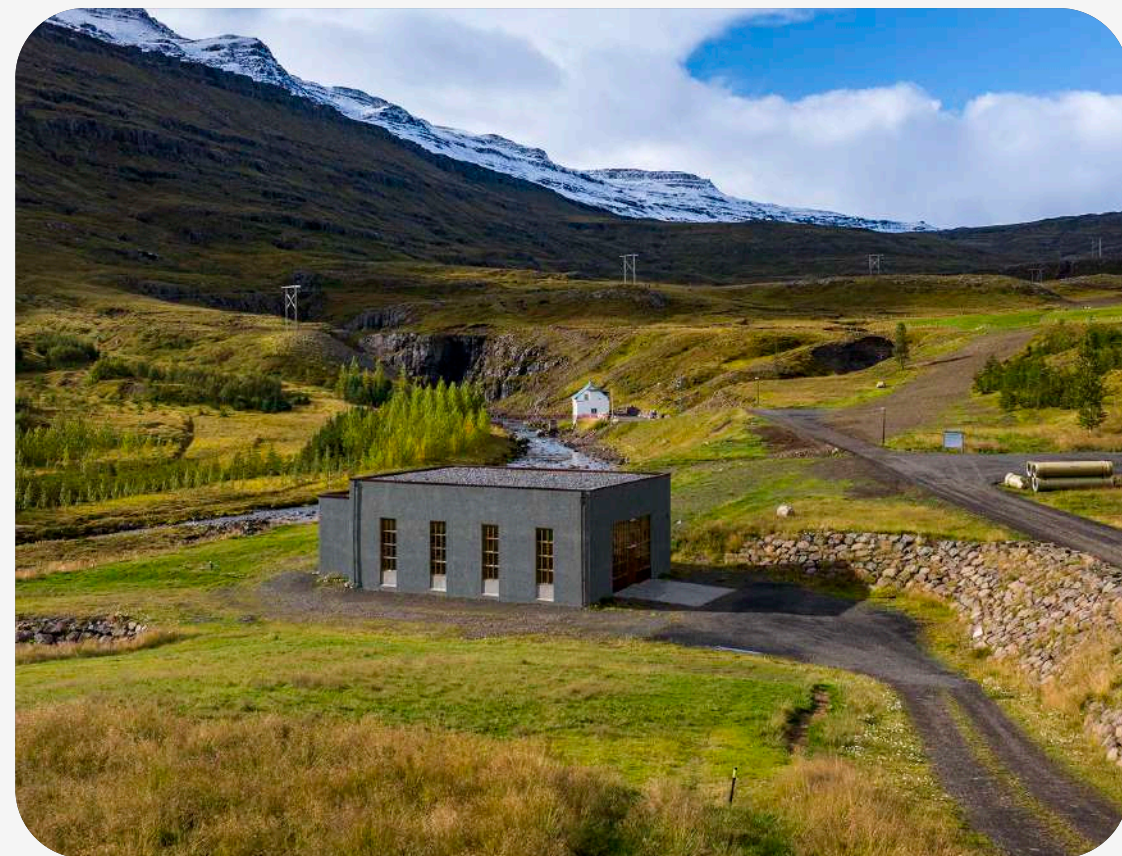
Bjólfsvirkjun in Seyðisfjörður is the downstream part of Fjarðarárvirkjanir.
